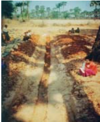
The sand in a riverbed has been removed and the 60 cm deep key has been excavated in the floor.
