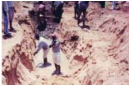
Two subsurface dams being build by self-help communities in Makueni, Kenya
