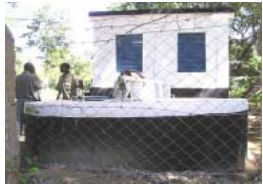
The completed well head with the pipe from the well to the pump.
