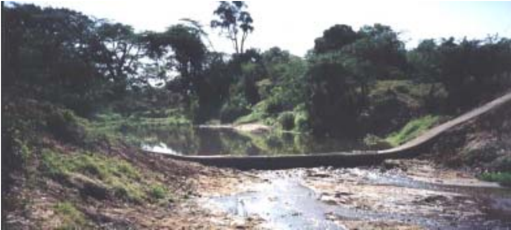
A weir constructed across Talek river in Maasai Mara was extended to be a sand dam to provide domestic water for a tourist camp. The lush vegetation seen upstream is due to the weir having raised the water table in the riverbanks.
