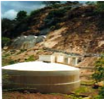
Rock catchment tank and dams.
