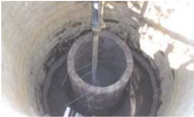
A small well shaft being sunk inside a wide well shaft of a river intake.
