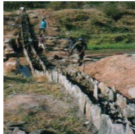
A subsurface dam being constructed of rubble stone masonry.
