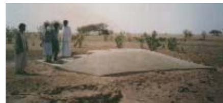
A hydro-dynamic well-head on a deep hand-dug well in a lugga.
