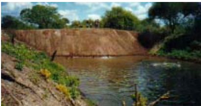
An earth dam built manually.
