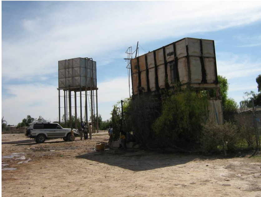
Figure 5-4: Two elevated tanks of the old water system in Erigabo
