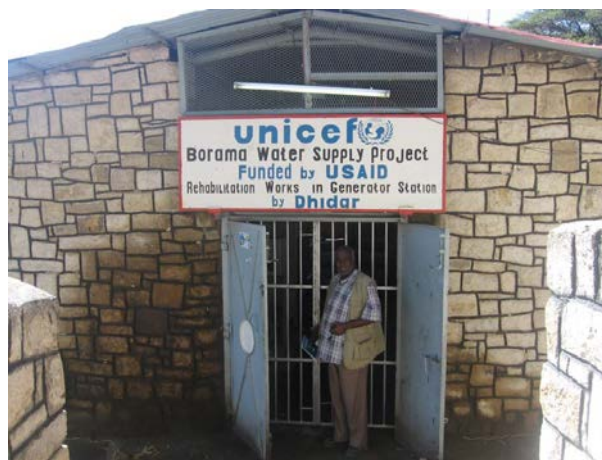
Figure 4-1: Generator station room for the Boroma water supply project
