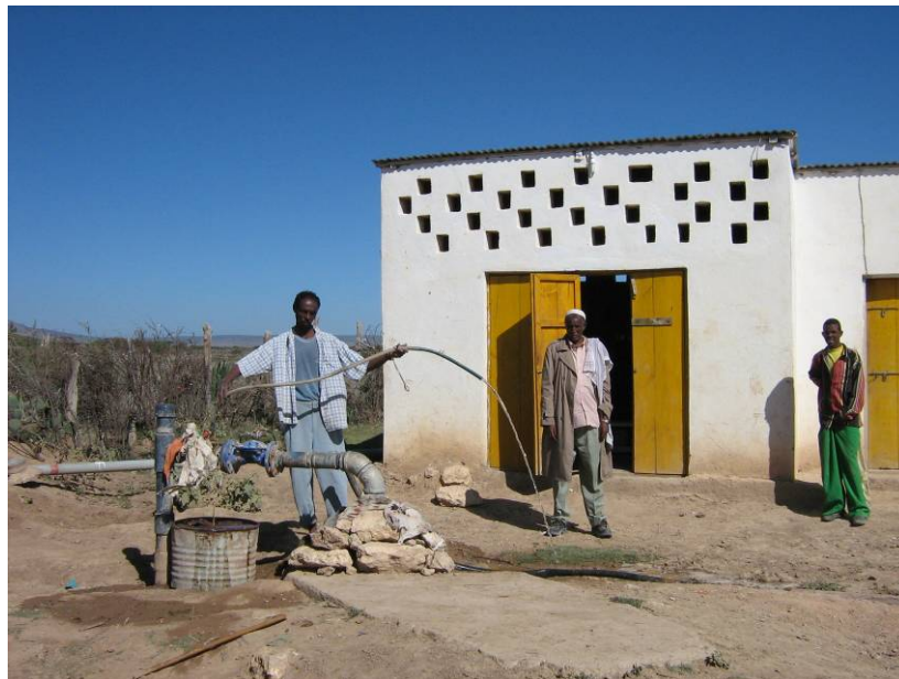
Figure 5-6: Recently-rehabilitated GTZ well No. 3 in Erigabo
