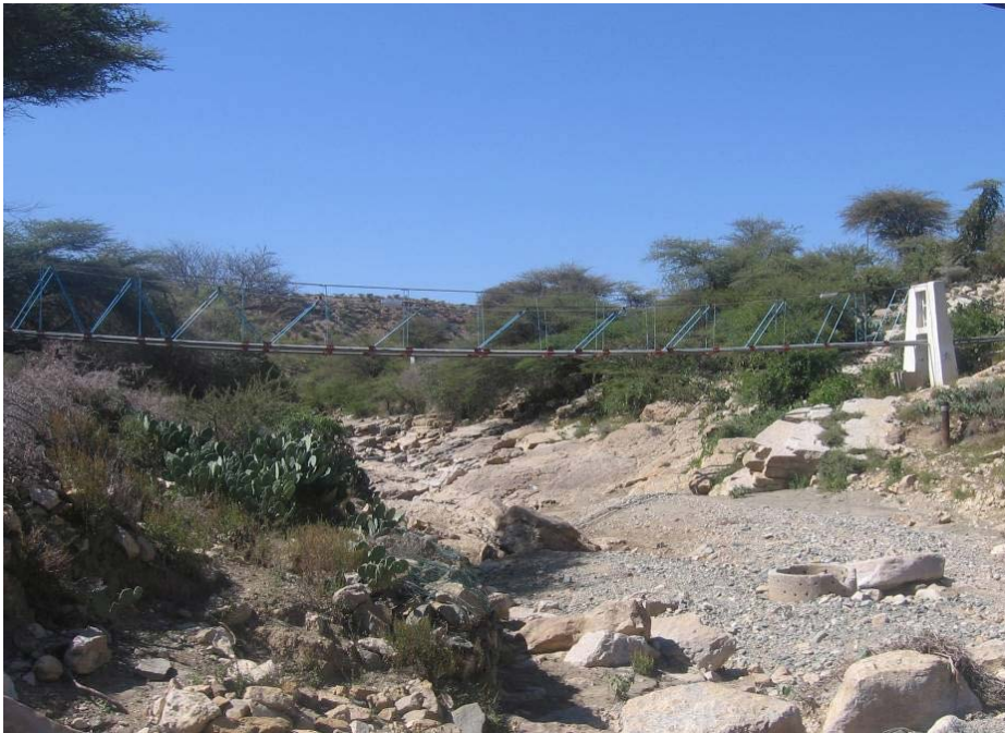
Figure 4-4: Suspension bridge, part of the piping distribution network system
