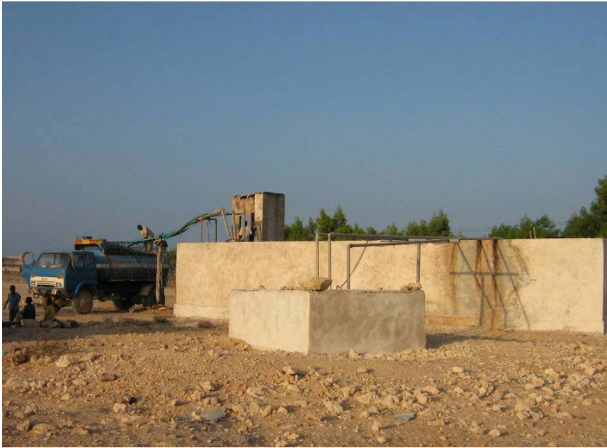
Figure 3-4: An example of privately owned tube well in the outskirts of Bossaso city
