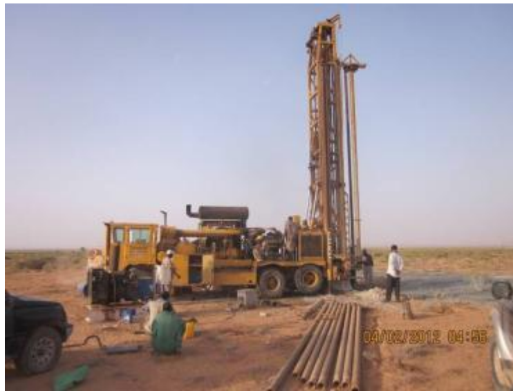
Figure 5.66 Drilling rig in operation in Toghdeer region (Photo Somaliland team 2)
