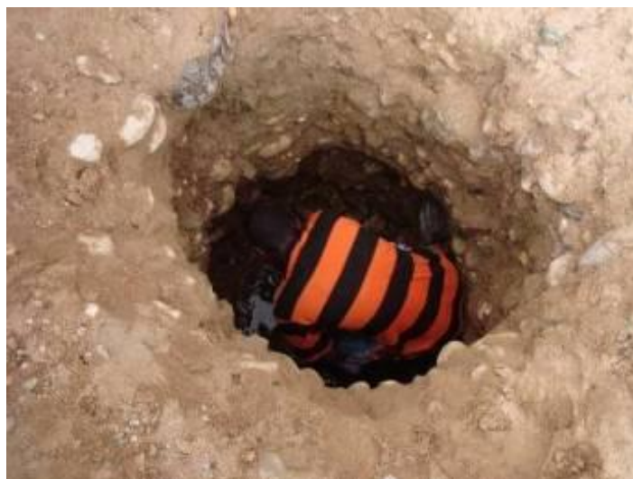
Figure 4.36 Very little water in well dug in Quaternary cemented carbonate crust (Photo of Somaliland team 2)
