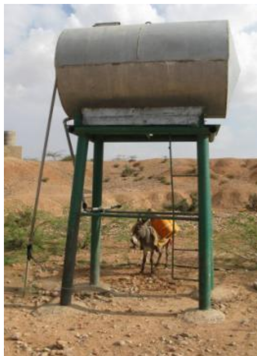
Figure 4.43 Water tank above the well tapping terrace Quaternary deposits near Jalelo (Hargeysa district, photo Z.Stevanovic)
