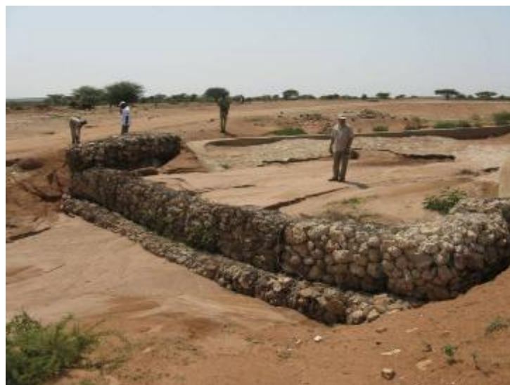
Figure 5.61 Gabions used as a barrier for sand dam (Woqooyi Galbeed, Somaliland, photo Z.Stevanovic)
