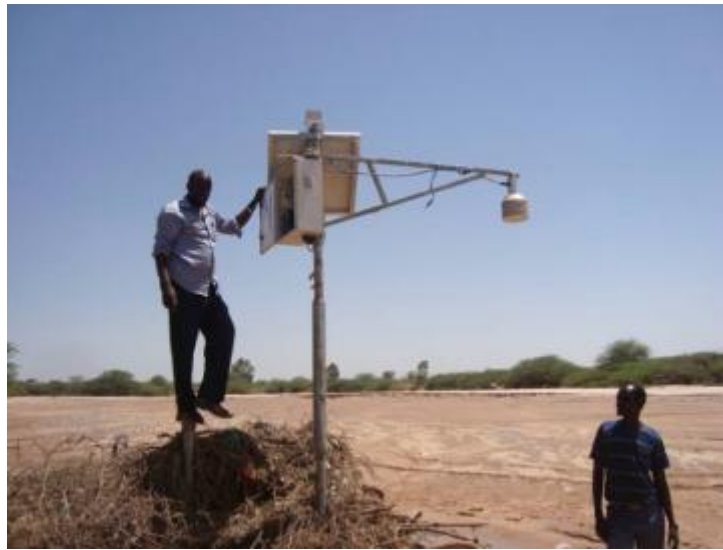
Figure 2.15 Installed automatic gauging station in pilot study area of Togga Waheen (FAO SWALIM)
