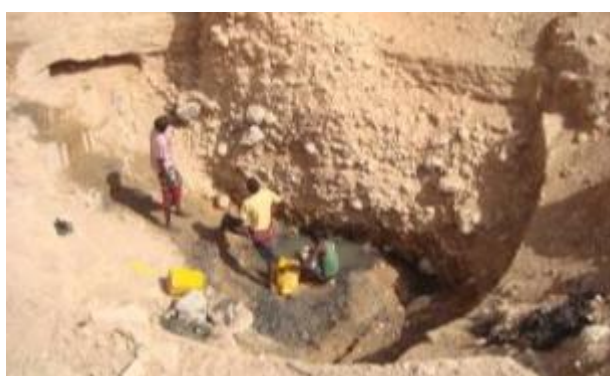
Figure 4.34 Excavated hole for utilization of small groundwater seepage
