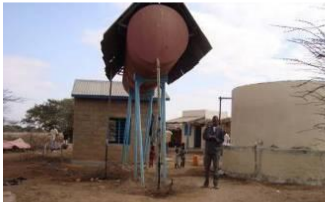
Figure 5.36 One of the wells and water tank in Borama area (Photo of Somaliland Team 2, Awdal)
