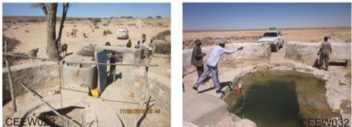
Figure 5.15 a,b Dug wells in the Sanaag region: CEEW 028,032
