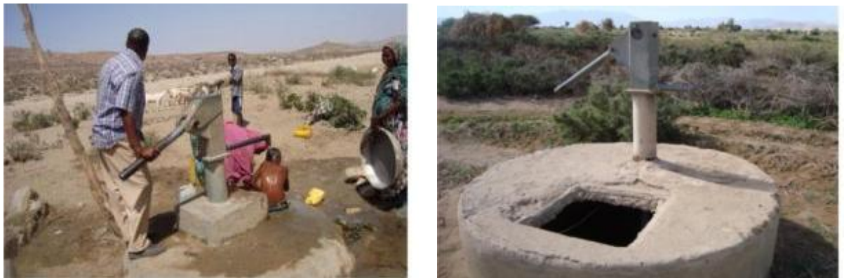
Figure 5.7 a,b Dug well BAW036 (left) and BAW039, with hand pumps
