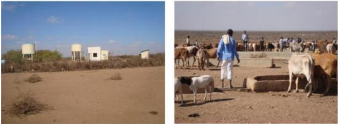
Figure 5.9 a,b Drilled well - GEB025 and use of pumped water
