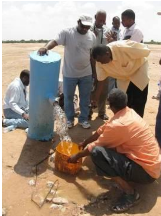
Figure 5.28 Recently drilled artesian well near Xunboweyle planned for Hargeysa new water source (photo Z.Stevanovic)
