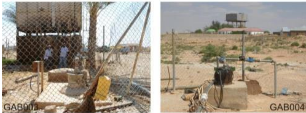
Figure 5.19 a,b Drilled wells in Nugaal region
