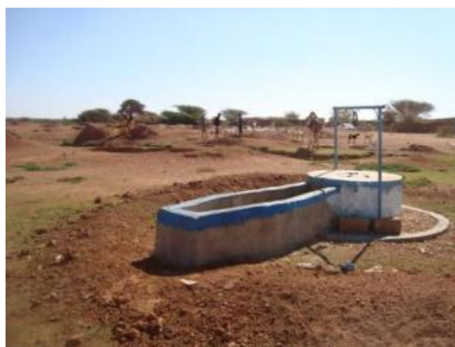
Figure 4.54 One of the shallow wells dug under humanitarian programmes in Somaliland to be used for humans but also for animals watering
