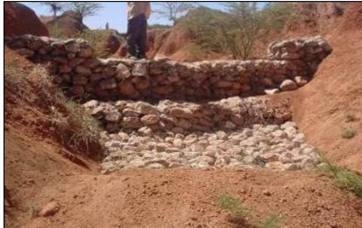
Figure 5.62 A small gabion barrier placed across togga in Durdur area (photo from German Agro-Action report, 2006)
