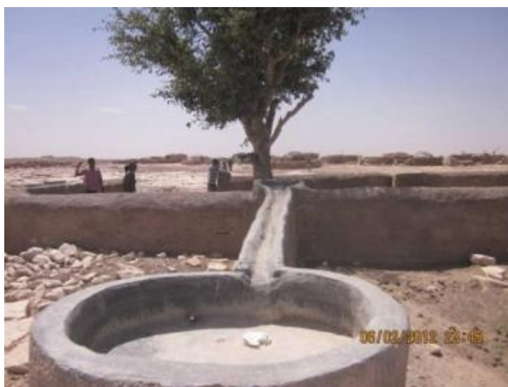
Figure 4.49 Dhabardalool shallow well in Ceel Afweyne area. Concrete construction is regularly includes canal for animals watering (Photo Somaliland team 2)
