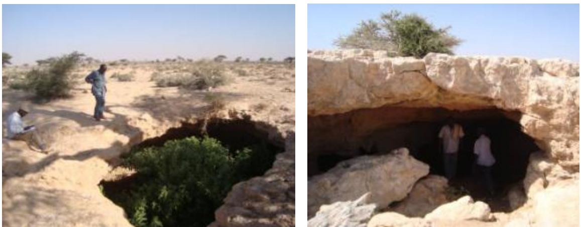
Figure 2.12 Collapsed roof of the cavern is creating a sinkhole (left, photo Puntland team) The cave carved in Karkar limestones (right, Buuhoodle area)
