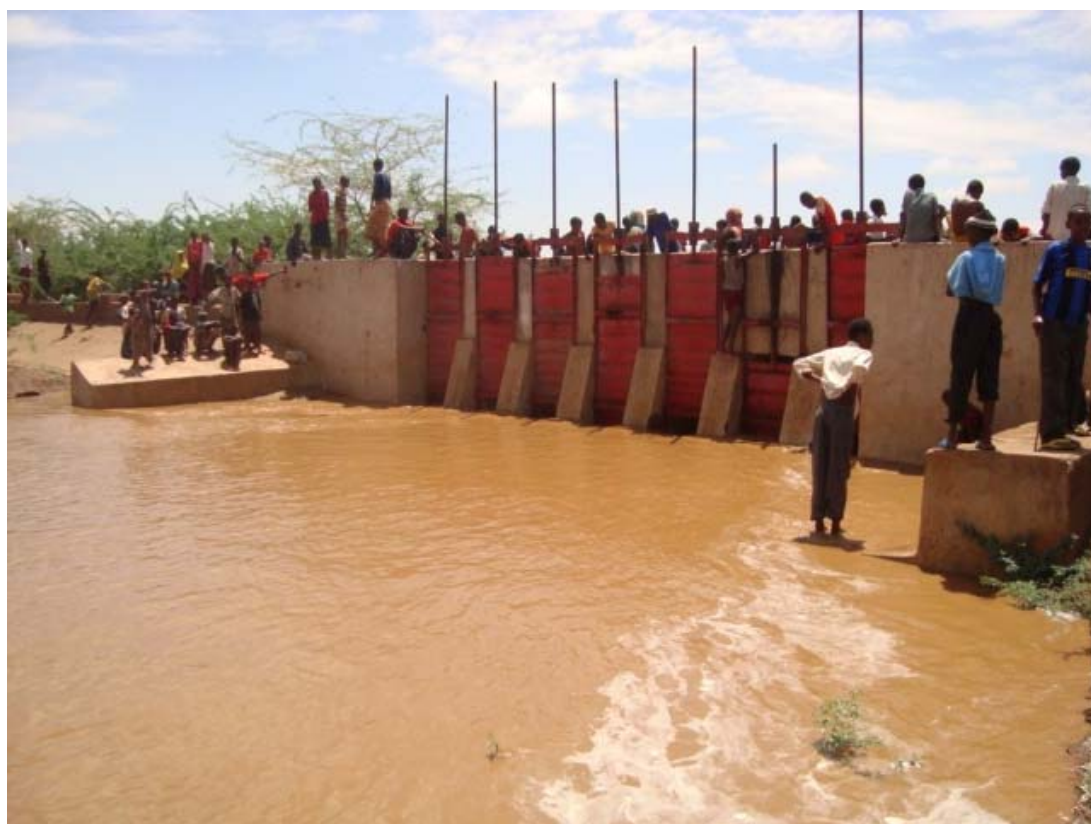
Figure 6.6: Photo of Belet Weyne Canal and Regulator
