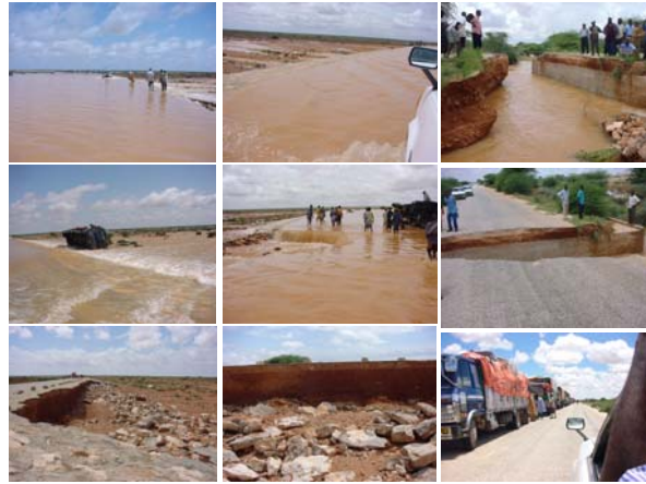
Figure 5.1: Impacts of May 2005 flash floods on a section of the Bossaso highway in the Puntland area 7
