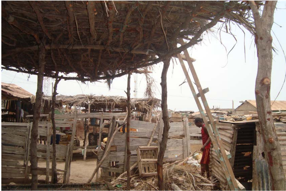
Figure 24: Construction by mangrove tree poles in Zeylac, August 2010
