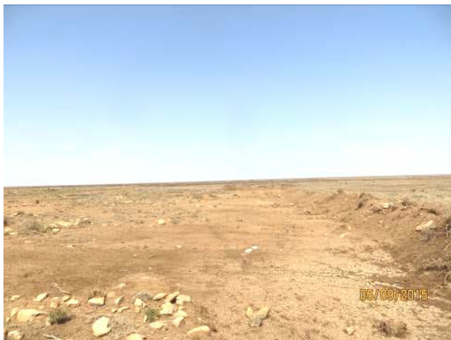
Soil bund constructed for soil and water conservation
