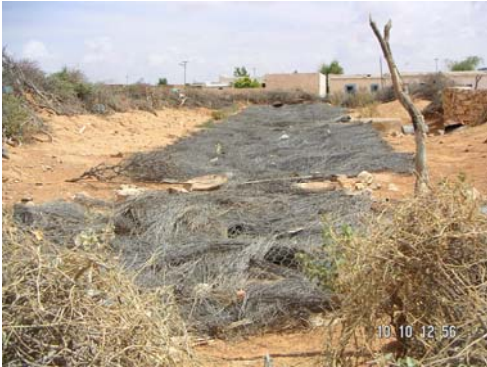
Oldest berked in the study area, located in Sherbi; dug in 1961 and covered with grass thatching
