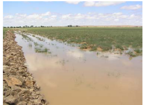
Rock dam after the rains detaining rain water and improving vegetation regeneration (Awsane Valley)
