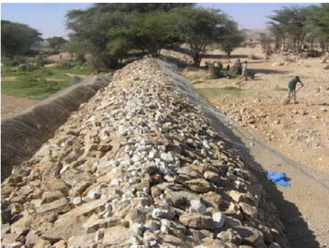
Check dam with gabion wire being put in place (Hadaftimo Gully)
