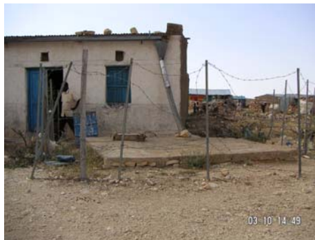
Oldest house berked in Carmaale, constructed in 1983
